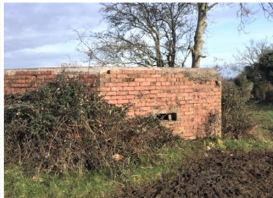
Type 29 Pillbox, Coal Pit Lane
