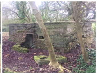
Type 29 Pillbox, Fry's Well Bridge
