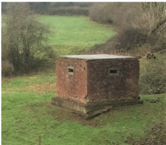
Type 26 Pillbox, Coal Pit Lane
