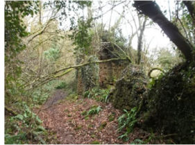
The remains of an old cottage
