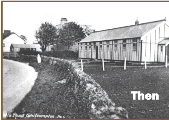
A view of Chilcompton Village Hall taken from the Wells Road
